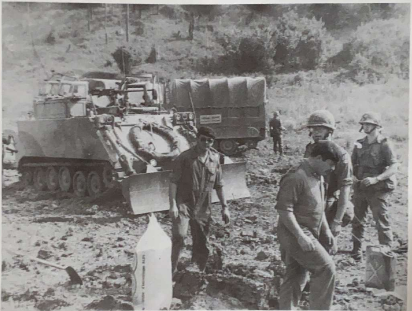
Engineer Demolitions. LCpls Smith & Wiffin making sure they don't get too involved RCH Hohenfels
