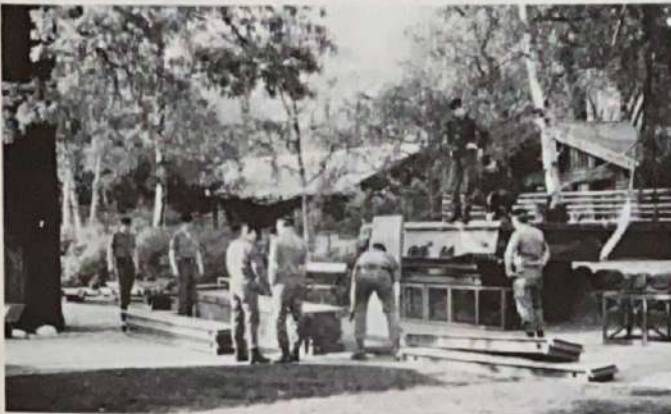
Building the bridge.
